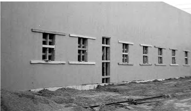
11.6b Bracing at Window Opening
