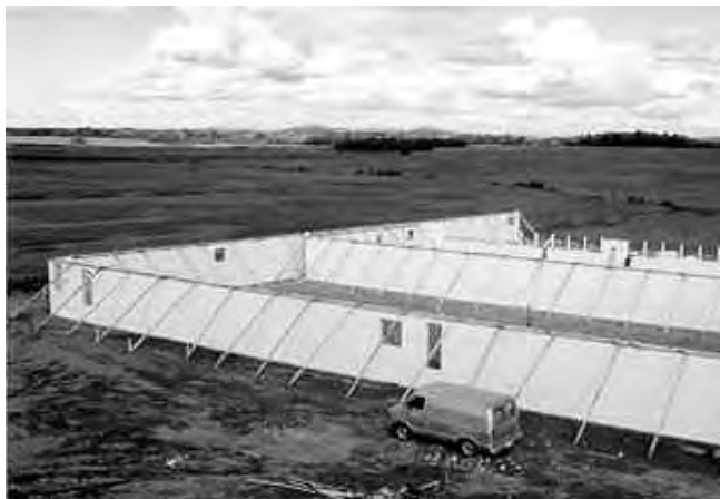
2.2 Bearing Wall Project in Progress
