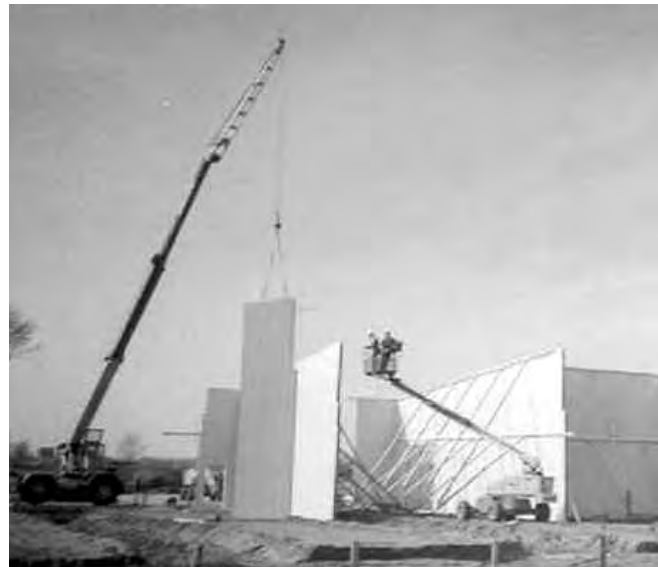
2.4b Erection of Pre-assembled Wall Section
