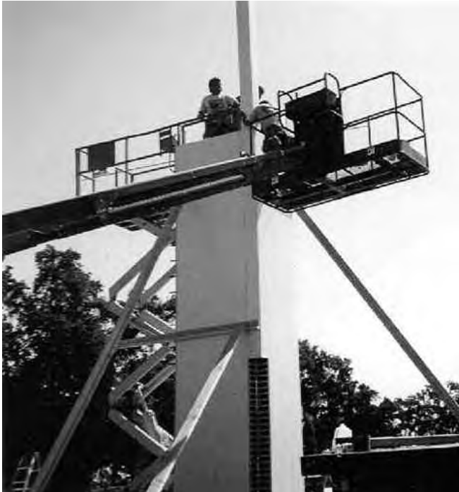
8.2a Erection of Conform Corner
