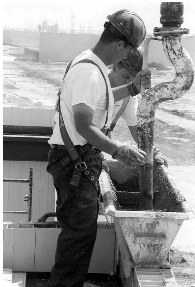
12.1b Concrete Funnel, Reducer and S-Bend
