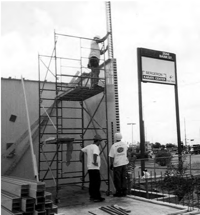
8.2b Erection of Conform
