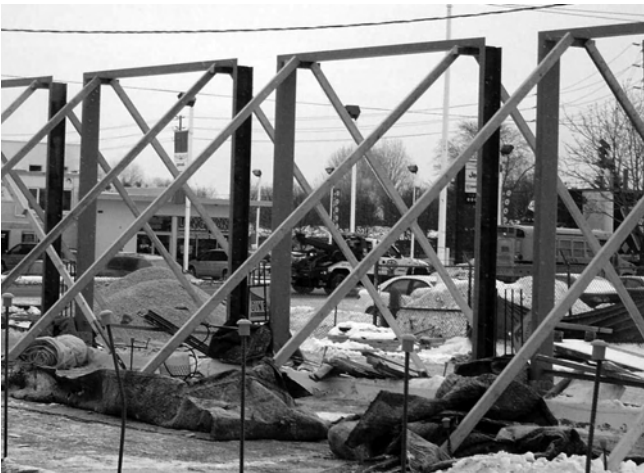
7.6a Overhead Door Frame Installation
