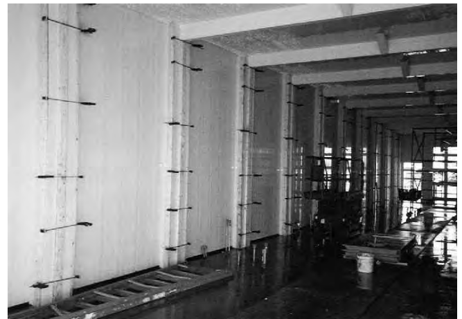
11.5d Bracing at Conform Pier
