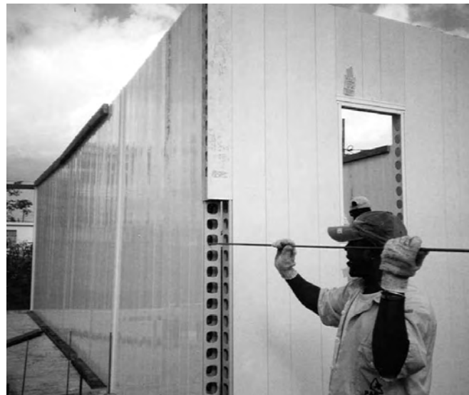
10.1b Horizontal Reinforcing Bars
