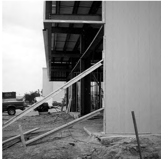
11.5a Bracing at End of Wall
