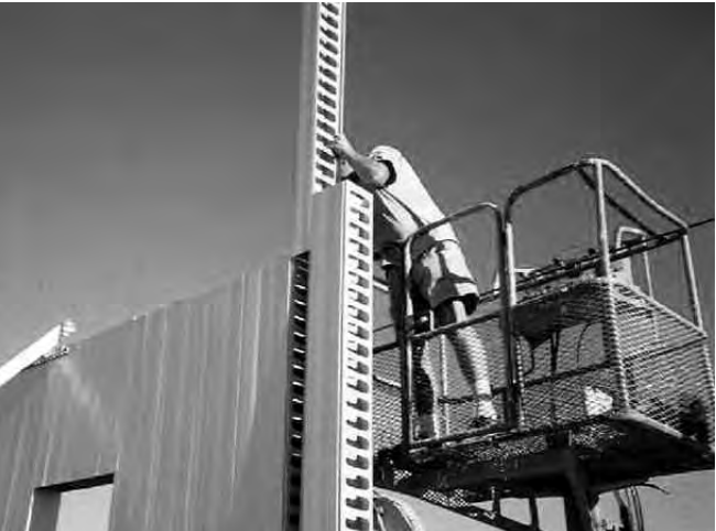
8.1 Erection of Conform Box and Panel
