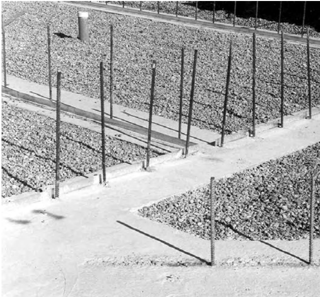
7.2 Metal Strapping and Dowels
