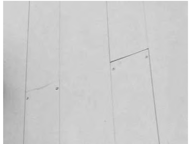
9.1b Screws at Staggered Joint
