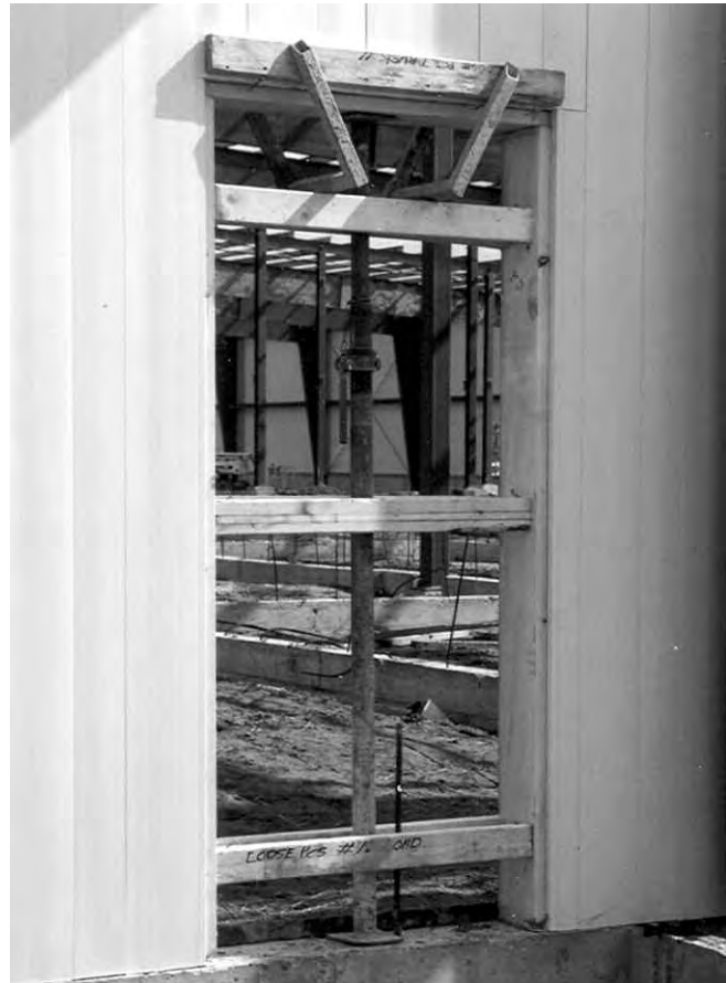
11.6c Bracing at Door Opening
