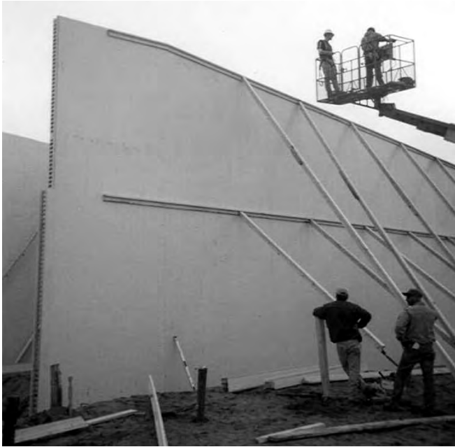
11.3a Mid Height Bracing at One Side
