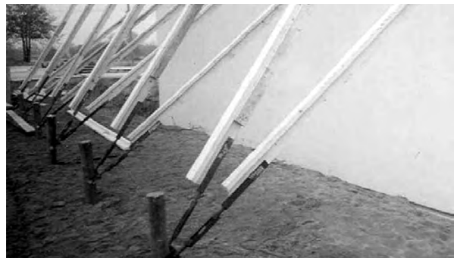
7.3 Wall Bracing and Form Aligners
