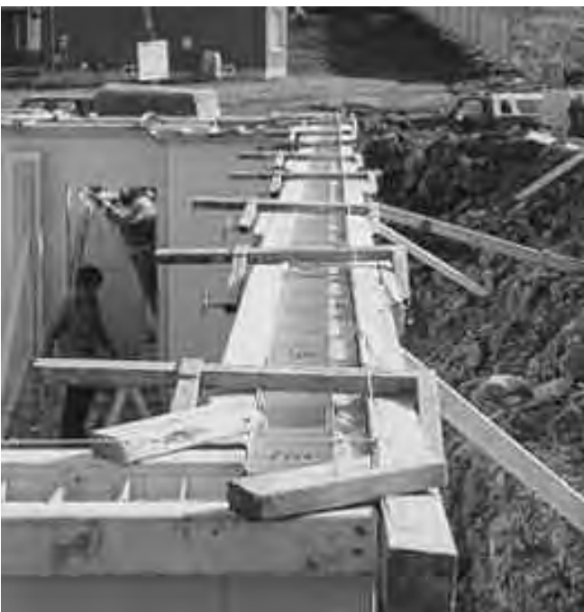
11.4b Top Bracing at Both Sides
