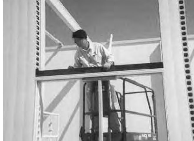
7.6b Steel lintel Installation
