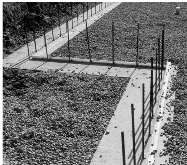
11.2a Bottom Bracing at One Side
