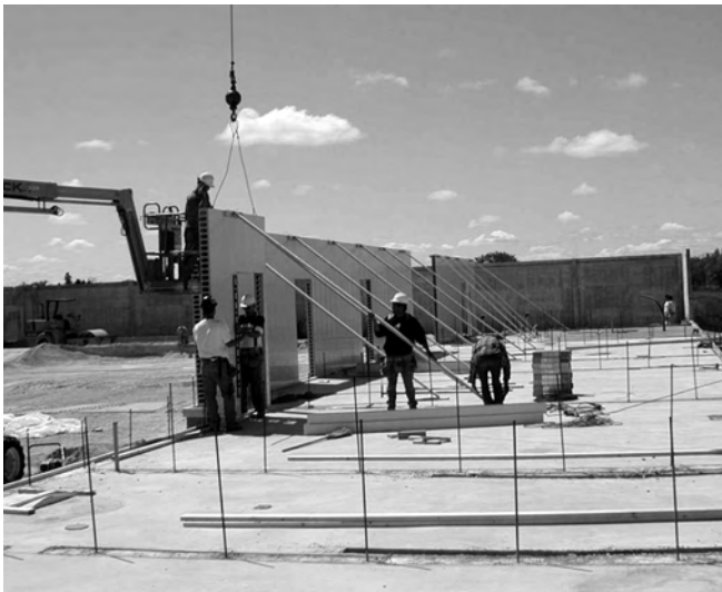
9.1c Pre-assembled Wall Section Lowered over Dowels
