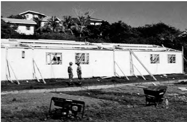
11.5c Bracing at Wall Intersection
