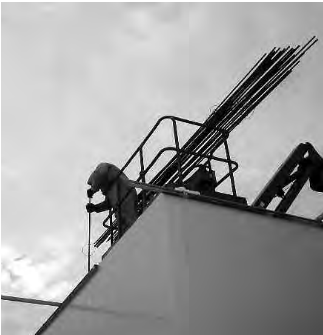
10.1a Vertical Reinforcing Bars
