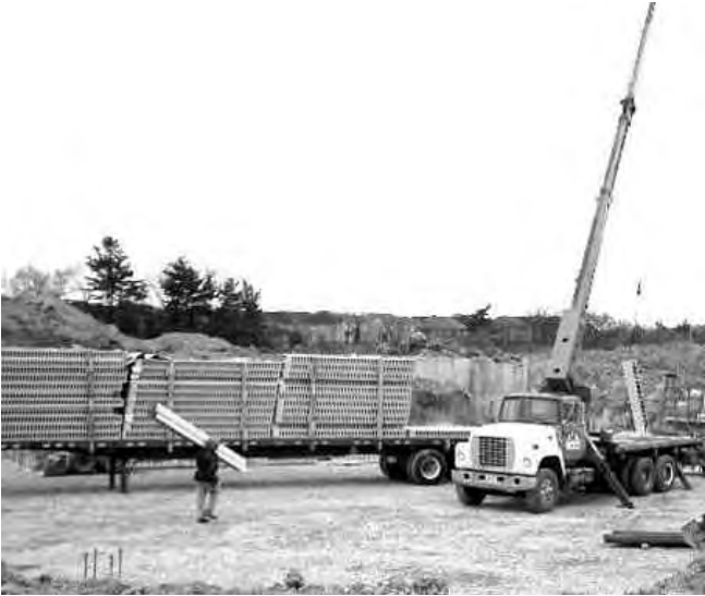
2.4a Pre-assembled Wall Sections for Off-Loading with Crane
