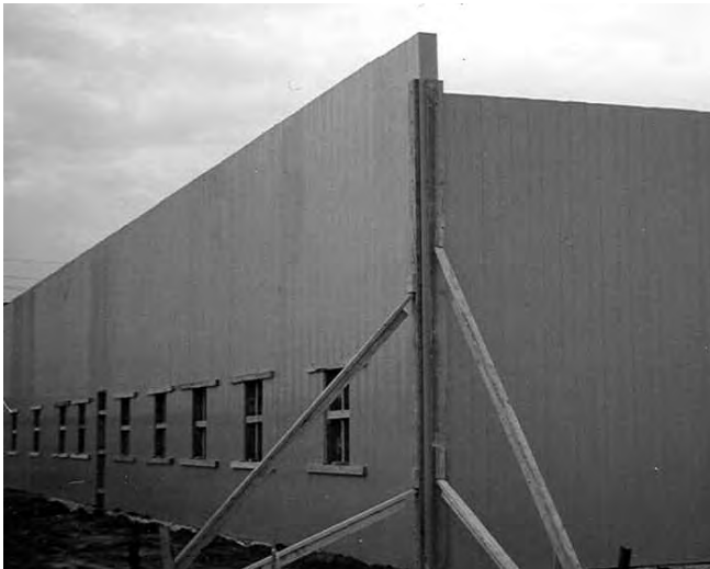
11.5b Bracing at Corner
