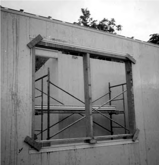
11.6a Bracing at Opening
