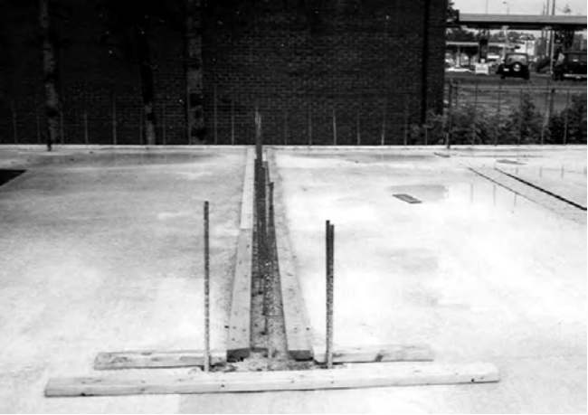
11.2b Bottom Bracing at Both Sides
