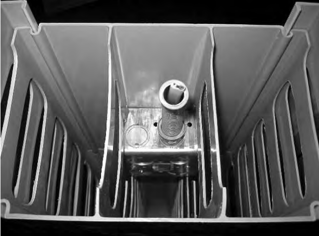
7.7a Electrical Box and Conduit
