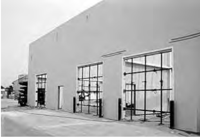
11.6d Bracing at Overhead Door
