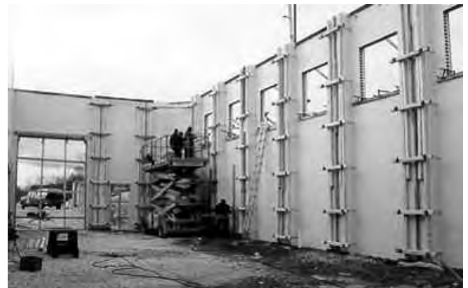
11.5e Bracing at High Pier
