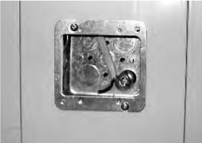
7.7b Electrical Box Installation
