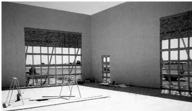
7.6c Bracing of Openings
