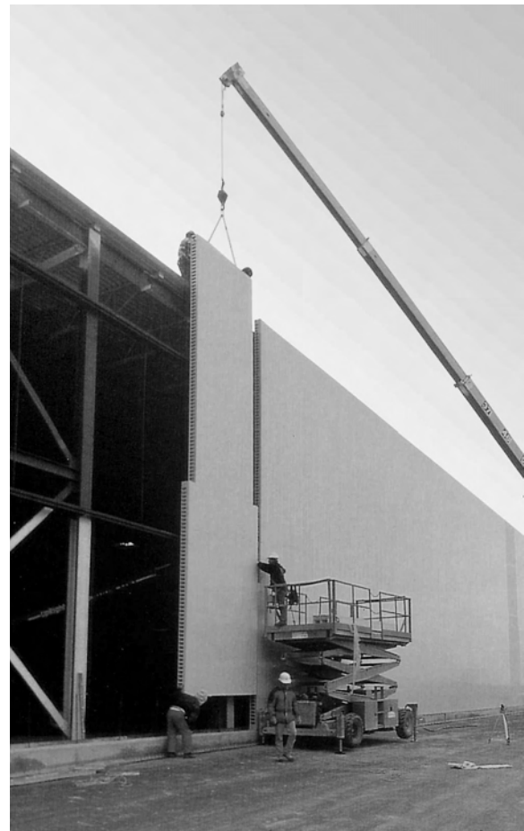
1.0 Non-Bearing Wall Project
