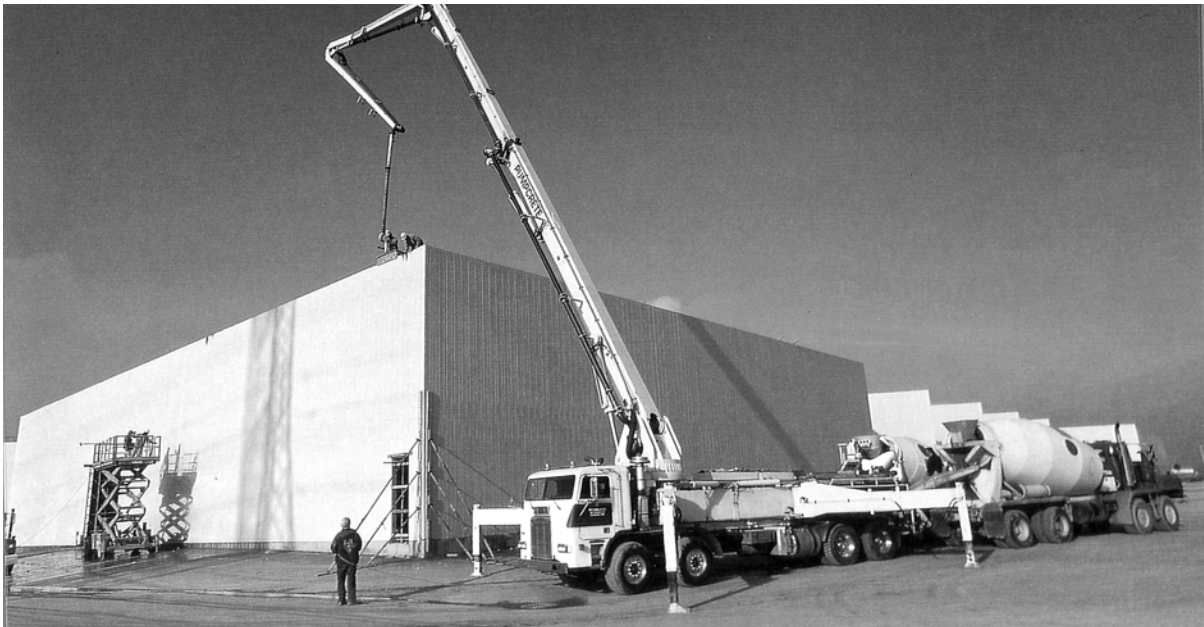
9.4c Concrete Placement
