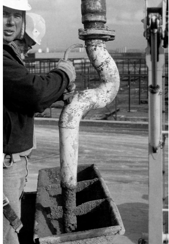
9.4a Concrete Placement
