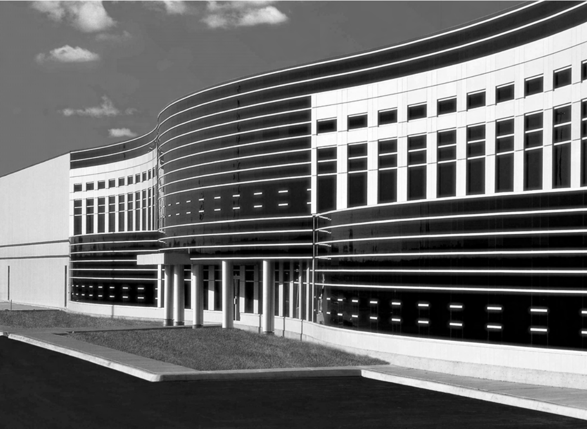
2.0 Completed Non-Bearing Wall Project
