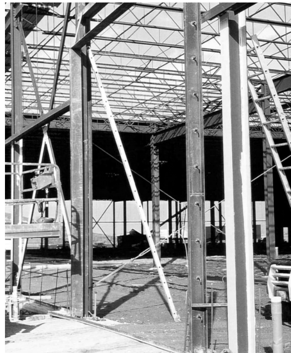
6.3a Structural Steel Framing
