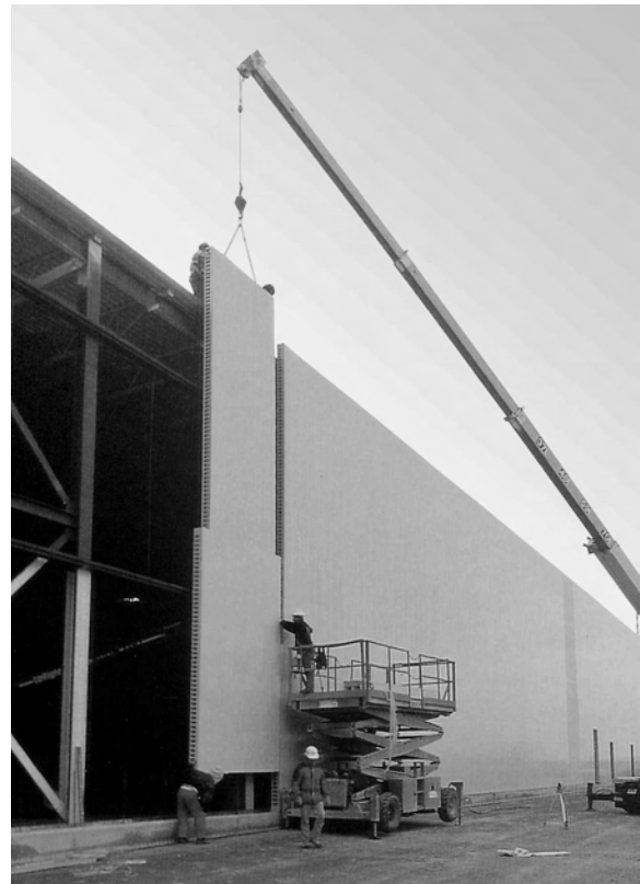
8.5d Pre-assembled Walls
