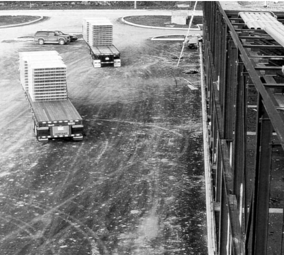
6.3b Structural Steel Framing
