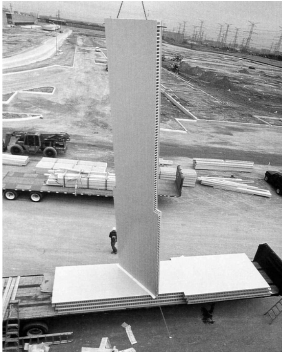
8.5b Pre-assembled Wall Sections
