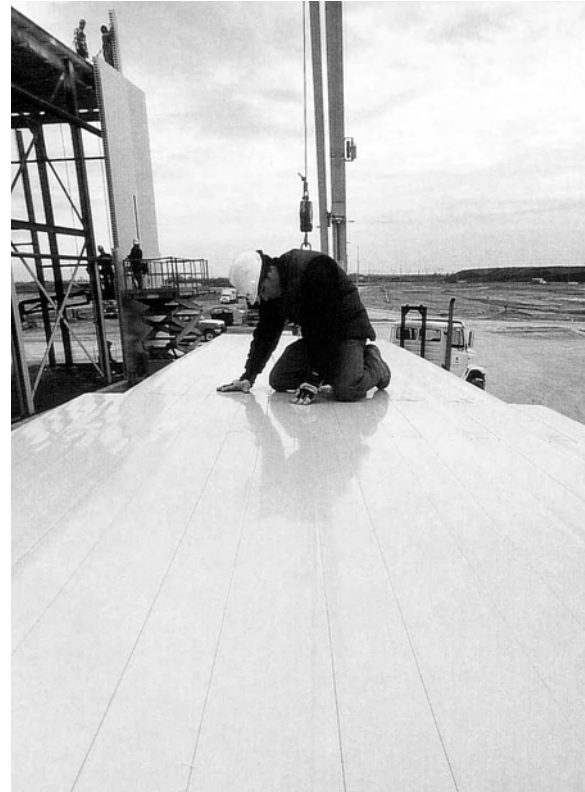
8.5a Pre-assembled Walls
