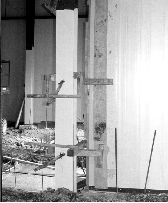
9.3b Wall Bracing & Formwork
