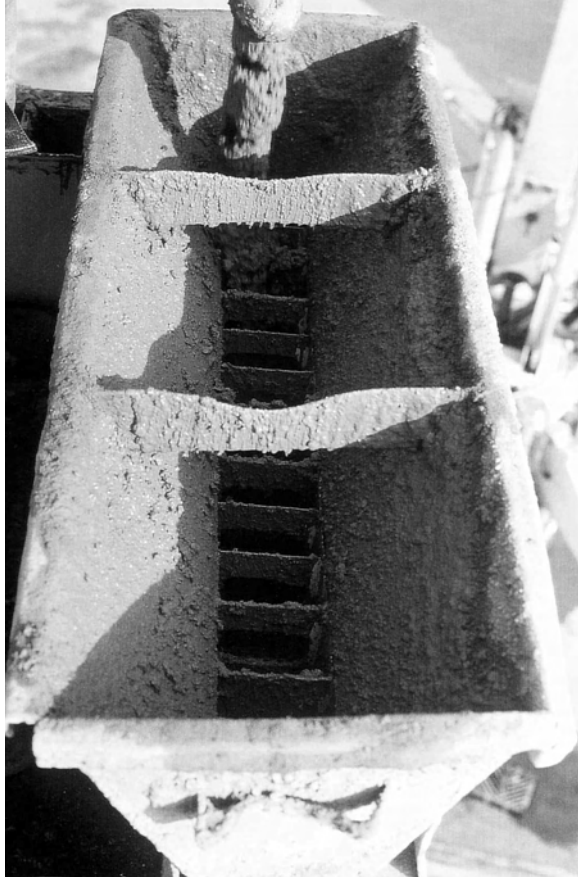
9.4b Concrete Placement
